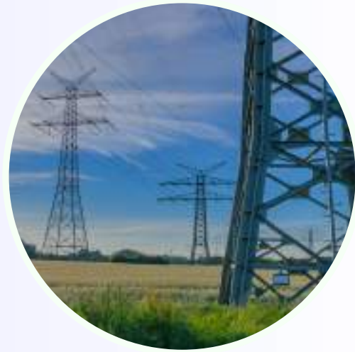
Electrical Power Generation & Transmissions
